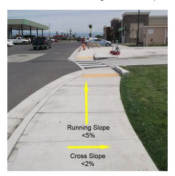
This here shows the running slope flat percent. The cross slope is maximum 2%. This references the problem I mentioned in Tallahassee with trying to push a wheelchair on the sidewalk that was so sloped, and in some places so steep, that I had to put all my weight on the inside of the wheelchair to keep it from flipping over.
