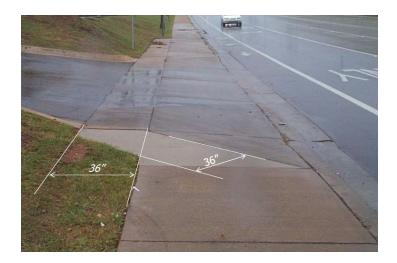
Now at a driveway apron, you have to provide a walkaround. If somebody is coming down the sidewalk in a wheelchair, or even somebody using a cane, a slope in a driveway can make it difficult, so you have to provide a 36-inch path and a 36-inch walkaround where the sidewalk is low.
