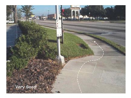
This image shows a well-constructed accessible route. There is a clear opening area in front of the traffic light controls for the crosswalk. There is a good accessible path.
